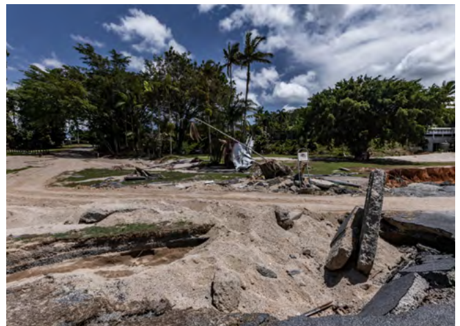
Destruction caused by Cyclone Jasper in Daintree Village.
